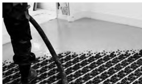
Flooding the underfloor heating system self-leveling mass.
