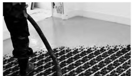
Flooding the underfloor heating system self-leveling mass.
