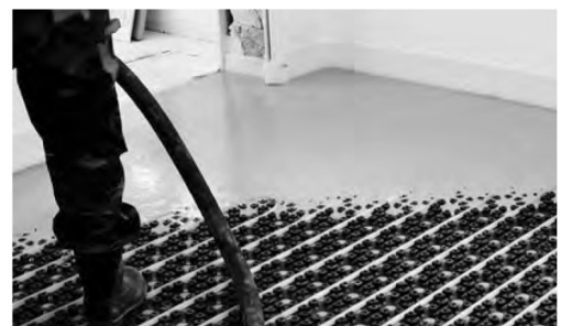
Flooding the underfloor heating system self-leveling mass.
