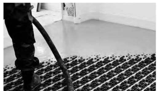
Flooding the underfloor heating system self-leveling mass.
