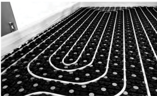
Underfloor heating installation with usage of EUROTOP Mini castellated mat.
